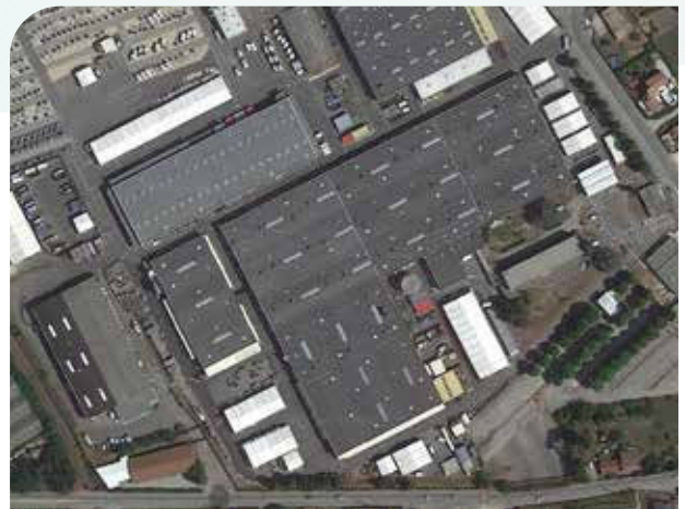
Aerial view of the Trigano site - Tournon-sur-Rhône
