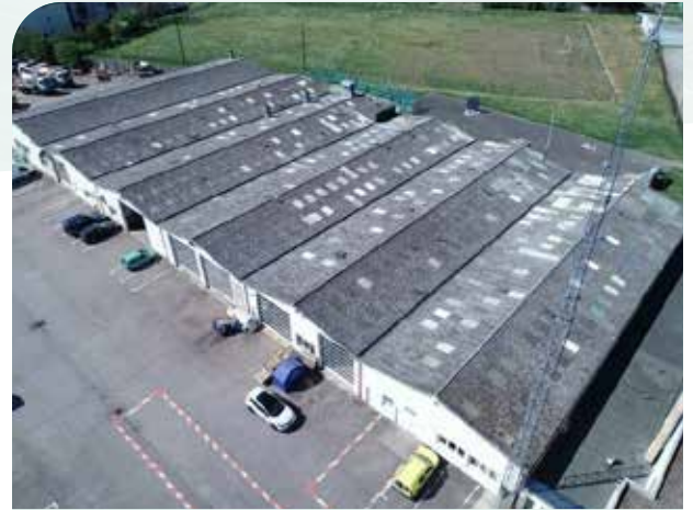
overview of the building before renovation
