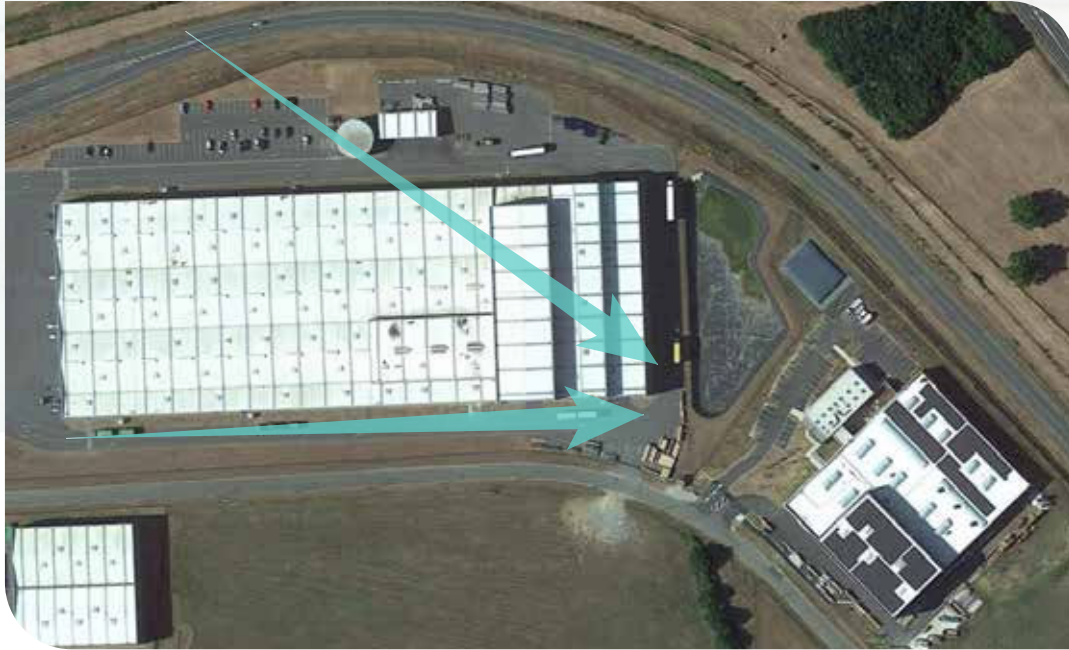
Masking effect of the neighboring building
