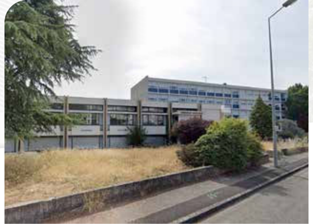
overview of buildings before renovation
